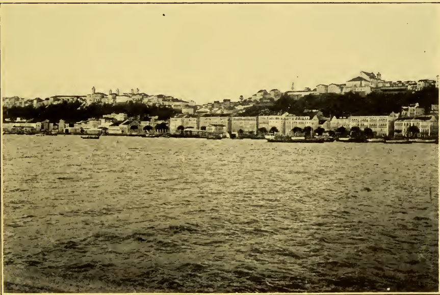
Partial Views of the City of Bahia from the Harbor.
